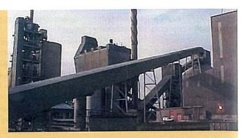
essentially comprised two sections of work. Firstly, to provide an enclosed independent clinker import station that would allow road vehicles to discharge and feed clinker onto the existing pan conveyor system feeding clinker store No 8. Secondly, to be able to divert clinker produced from No 7 kiln into a rejects silo from where it could either be conveyed, by a new pan conveyor, to the No 8 clinker store or loaded to road vehicles, in an enclosed facility with a second clinker import station.
