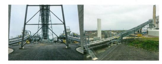
The intermediate storage silos hold the pellets prior to them being fed into 12 individual dense phase conveying systems to reach the grinding mills that will pulverise the pellets before being injected into the boiler burners. Lynemouth has three boilers and each is served by four mills each of which has four dedicated dense phase conveying systems, one of which is a hot standby
