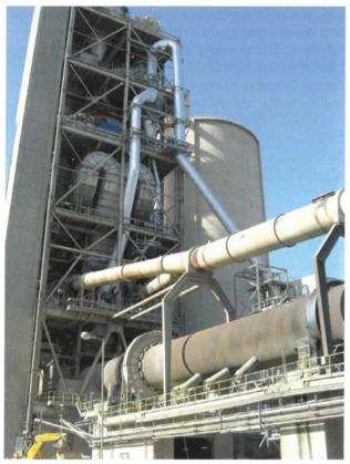
Kiln bypass at Ketton cement plant.
